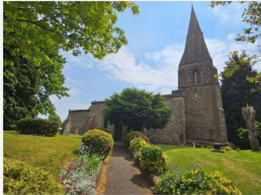
Figure 15: St Michael's Church, Diseworth– Grade II* Listed
